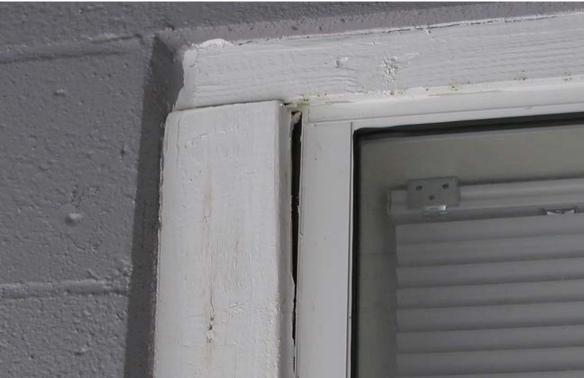
Instances were noted where damaged or deteriorated wood was not replaced or repaired prior to painting rehabilitated homes.
