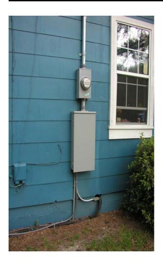
One client expected the breaker box that was inside of her home previous to the rehabilitation to be reinstalled in the same location. The contractor relocated the breaker box outside of the home during the rehabilitation without consulting the client. The client feels that the breaker box outside of her home is difficult for her to access as she is handicapped and uses a wheelchair.
