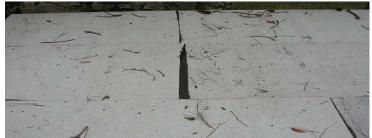
Roof seams were not properly spaced (i.e., offset).
