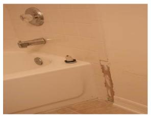
Tile was missing in several places in the master bathroom. The tub did not drain and was not functional at the time of our site visit on February 13, 2008. The homeowner indicated that the master bathroom tub had not drained since the completion of her home rehabilitation.
