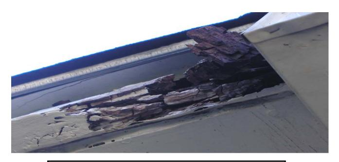
The wood around this replaced roof does not appear to have been repaired or replaced prior to painting. The final payment was made on this project on July 17, 2006, approximately 15 months prior to our site visit.
