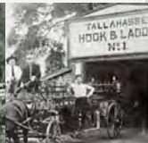
First City Fire Station
